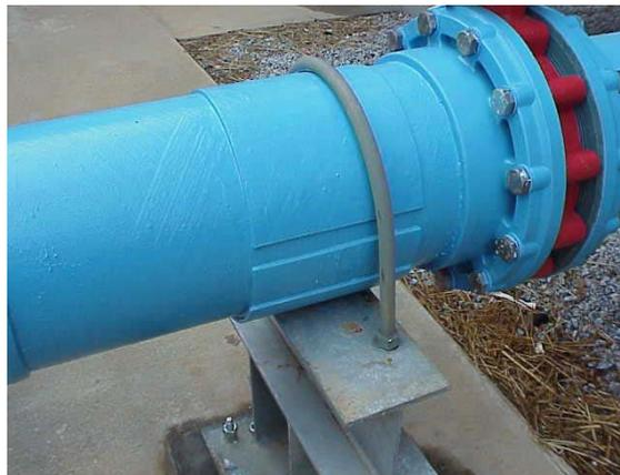
*Figure 8.1-4 U-Bolt Arrangement*
