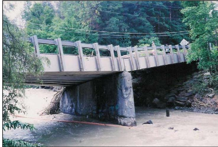
*Figure 9. Damaged County Route 1 Bridge over Van Campen Creek.*
