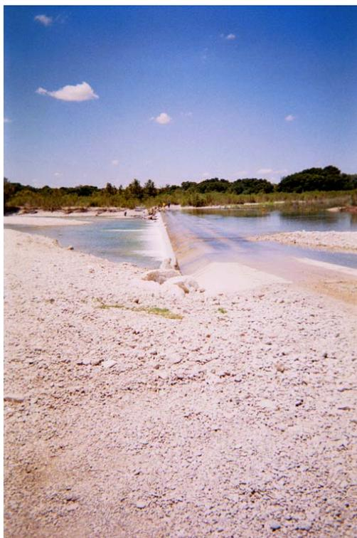
Figure 4. Typical concrete slab low water crossing (without pipes).
