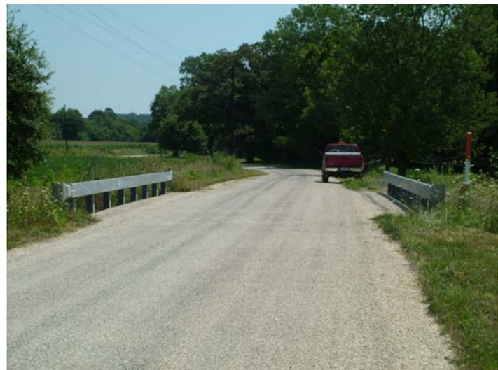
*Figure 9. New Belleview Hollow Road Bridge – widened road and shoulders.*
