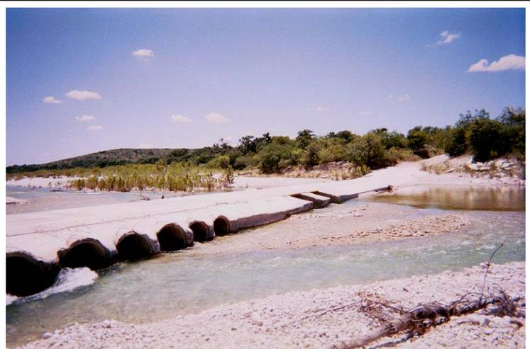
Figure 5. Typical concrete slab crossing (with pipes).
