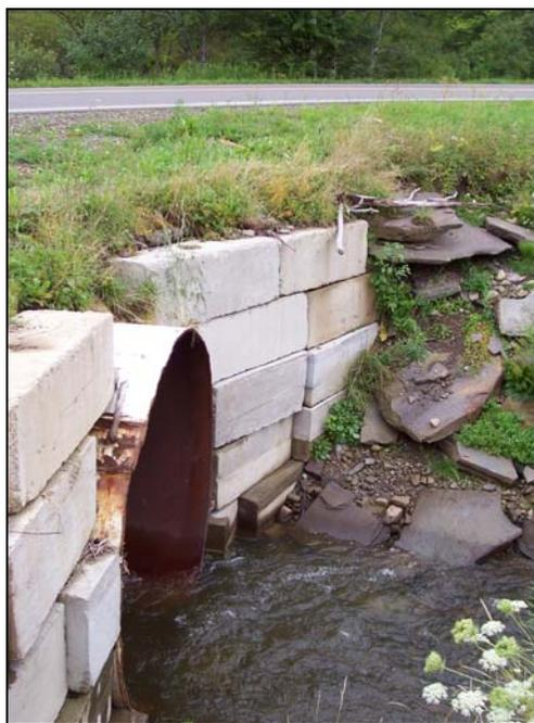
Figure 6. Temporary headwalls at railroad tank culvert
