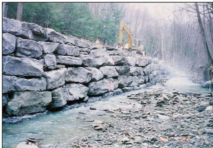
*Figure 8. Stone stream bank protection*
