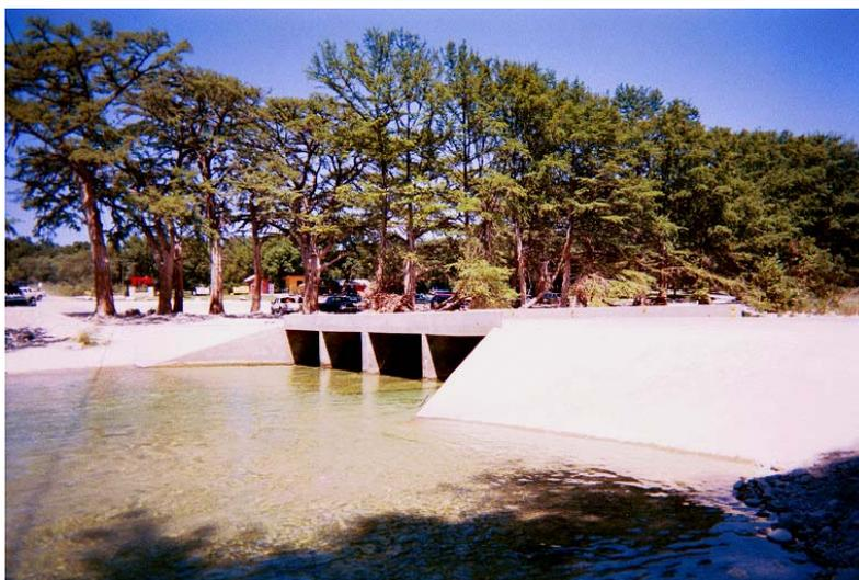
Figure 10. Typical box culvert built by Uvalde County, County Road 348 over the Frio River.
