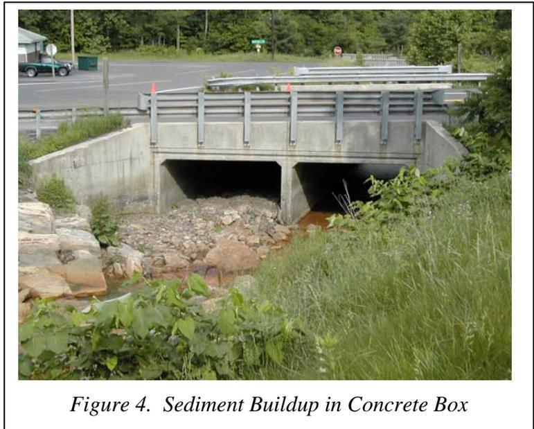
*Figure 4. Sediment Buildup in Concrete Box*
