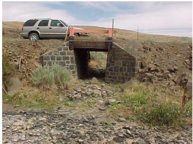
Figure 3. Outlet of Typical Short Span Bridge
