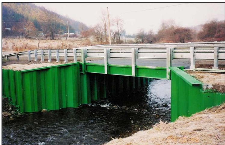
Figure 5. Typical small bridge built by County's crew
