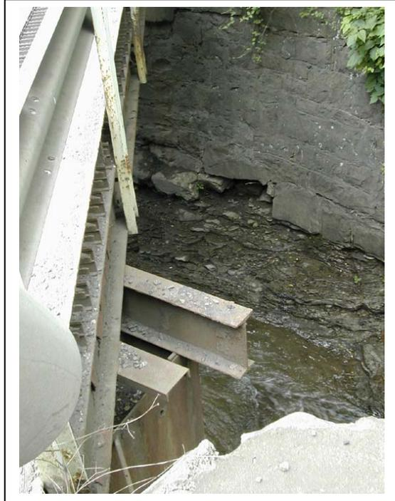
*Figure 7 and Figure 8. Deteriorating Abutments*
