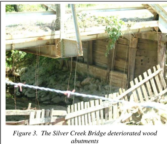
*Figure 3. The Silver Creek Bridge deteriorated wood abutments*
