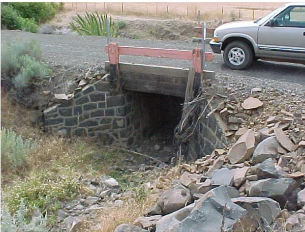
Figure 2. Inlet of Typical Short Span Bridge
