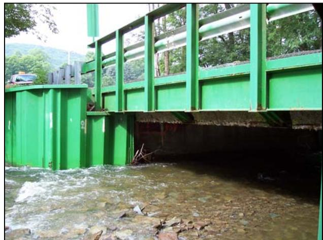
*Figure 7. Sheetpiling improves inlet conditions*
