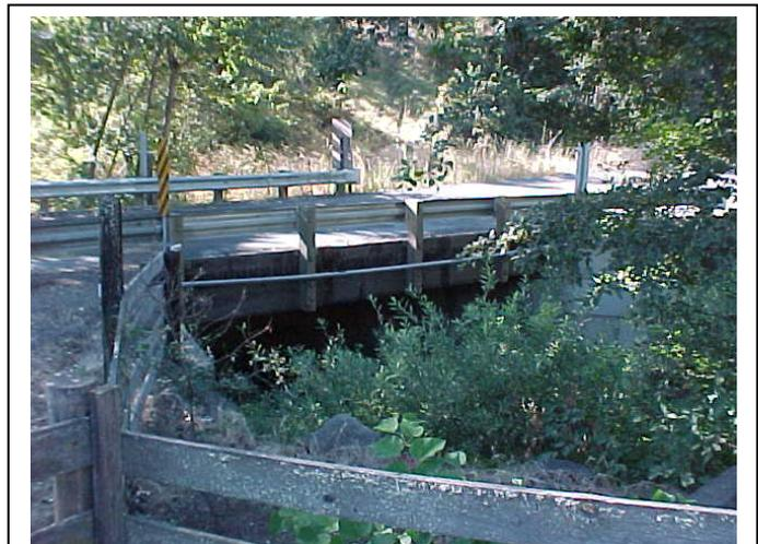
*Figure 6. Upstream of Bridge 65C74 (timber superstructure, concrete abutments, vegetative growth in stream)*
