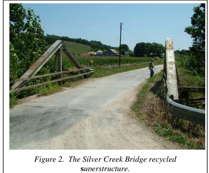
*Figure 2. The Silver Creek Bridge recycled superstructure.*
