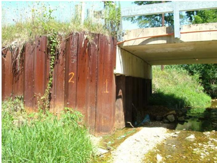
*Figure 8. Metal sheetpiling at Belleview Hollow Road Bridge.*
