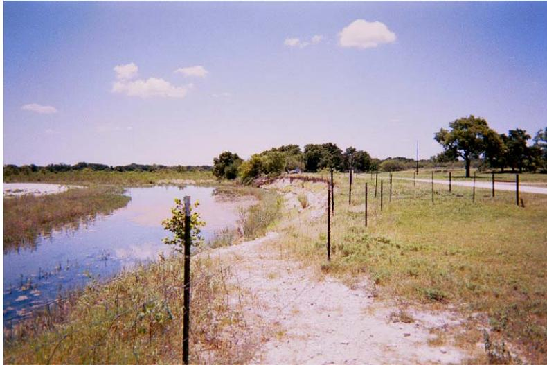
Figure 9. High bank erosion threatens relocated unpaved road (to right).
