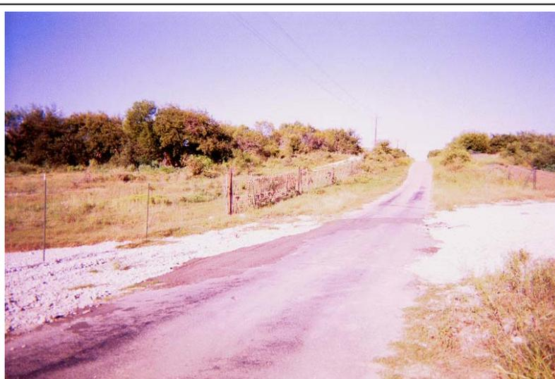
Figure 8. Typical dip in unpaved road, showing washout path (from left to right).
