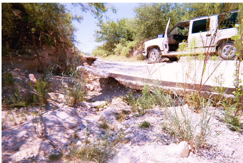
Figure 11. Scour at transition of approach road and crossing.
