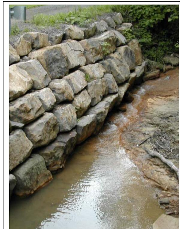
*Figure 5. Installed Imbricated Riprap*
