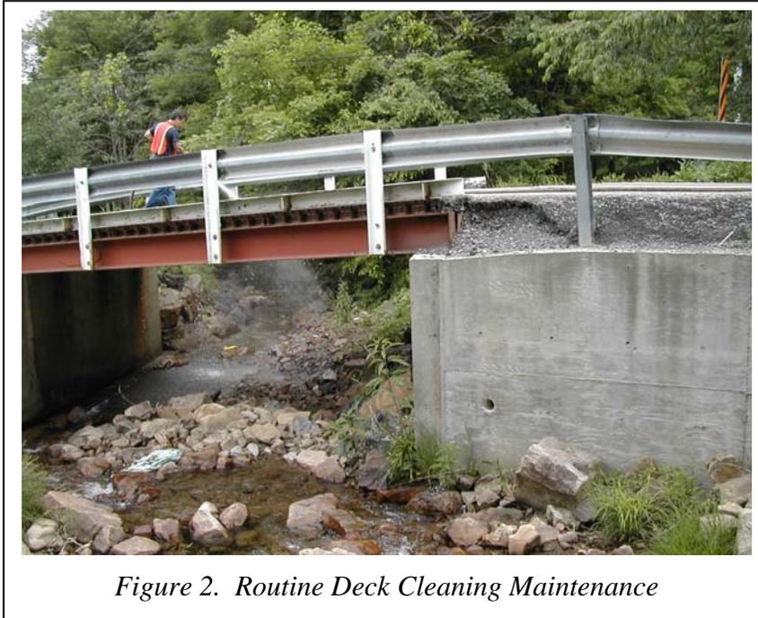
*Figure 2. Routine Deck Cleaning Maintenance*
