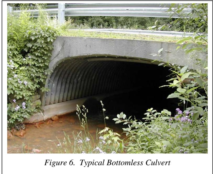
*Figure 6. Typical Bottomless Culvert*
