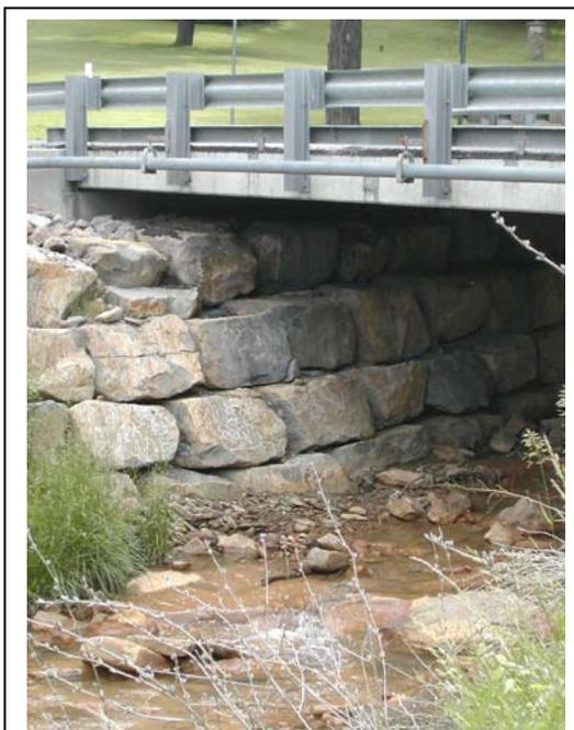
*Figure 10. Sugar Maple Road Imbricated Riprap Protected North Abutment (looking upstream)*
